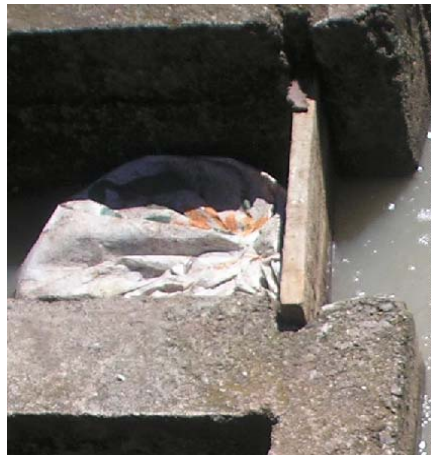
Figure 9 Control Gate Installation in Imhoff Tank
